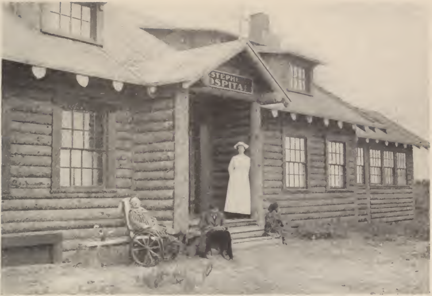
OUR NEW HOSPITAL AT FORT YUKON
